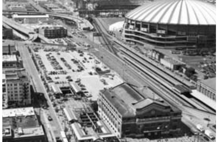
Union Station Development after underground garage construction. Structures to the left of Union Station are entryways to the bus tunnel.
